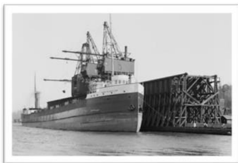
1906-At the Copper Range Coal Docks
